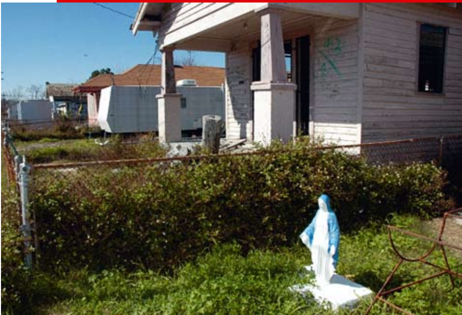
Abandoned houses in New Orleans after the hurricane Katrina. LA. 2007, 2008
